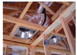
Jump ducts allow air pressure between rooms to equalize through the ductwork.
